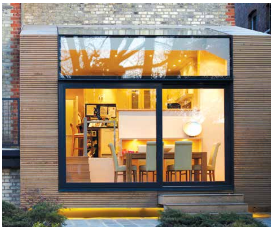
The façade of the extended house on Church Crescent (photographs by Janie Airey)
