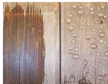
Untreated Cedar wood exposed for 18 months (left) and treated with Manalox WB10 (right)
